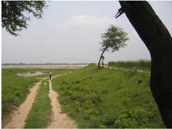
Embankment and river in the distance
