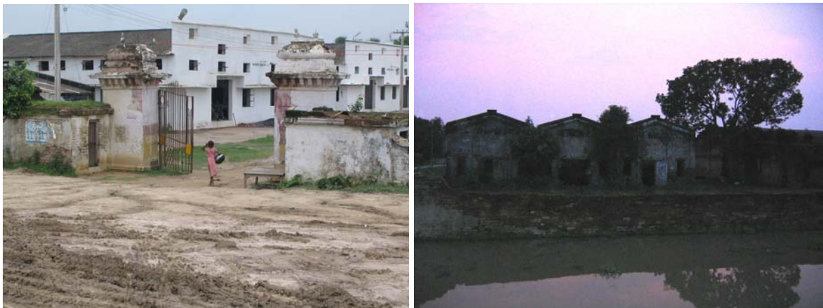
Defunct industrial units
